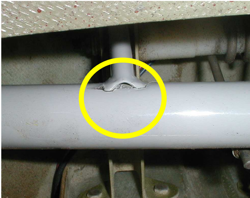
picture 3: Damage viewed from front
